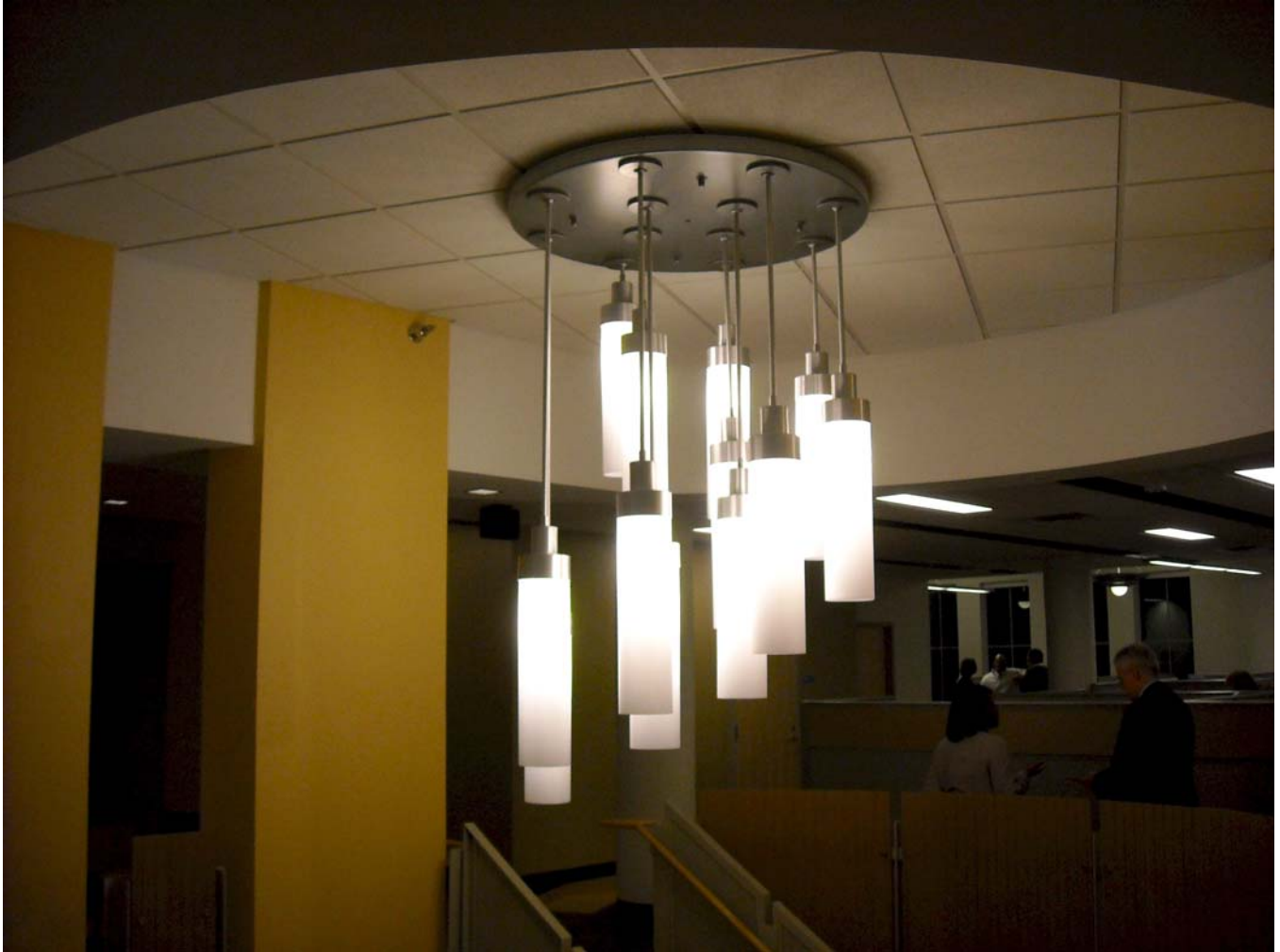
Brushed Aluminum Finish with Painted Aluminum Canopy Satin White Acrylic Cylinders 48" Diameter, Each Cylinder 28" Body Height, 78" Overall Height Lamping – 12 CF-26 GU24 Base 120V
