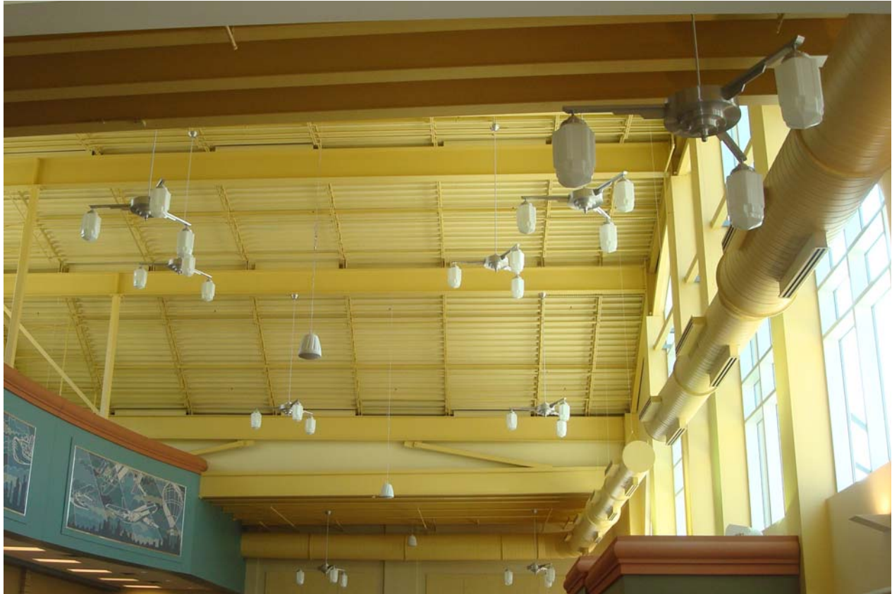
Brushed Aluminum Finish 10" Diameter White Opal New York Glass 72" Diameter, 26" Body Height, Various Overall Heights Lamping – 3 250W ED28 Pulse Start Metal Halide 120V
